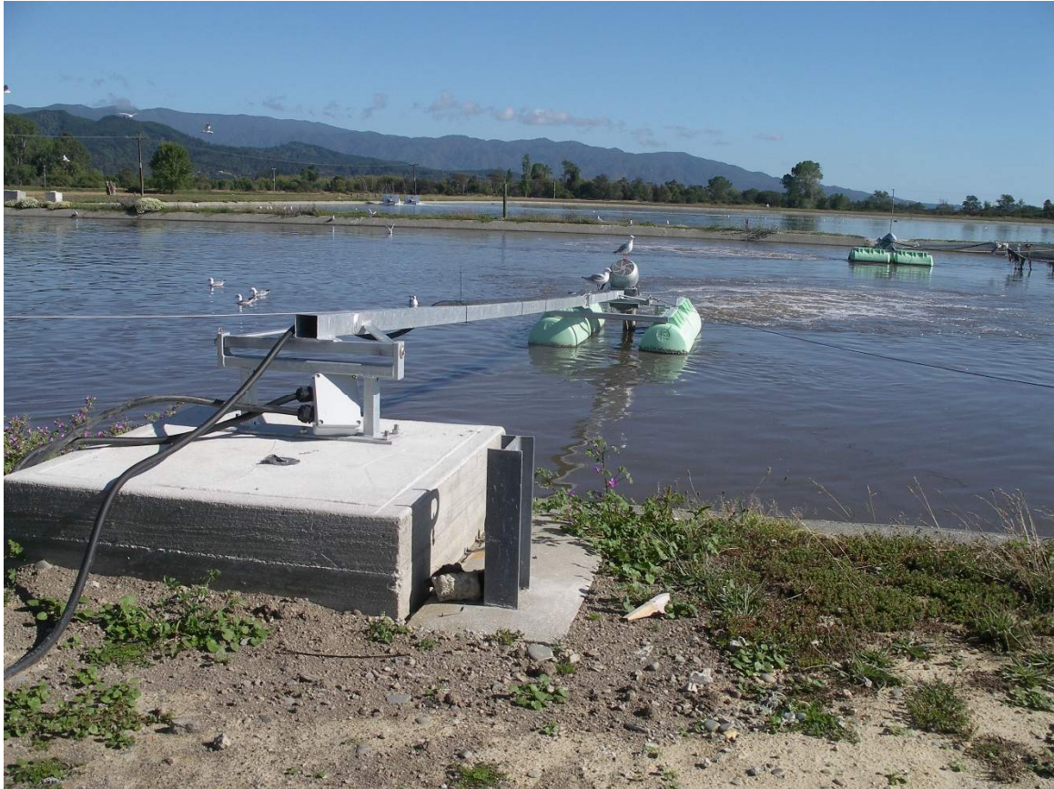
Photo 3: New directional aerator on Pond 1
