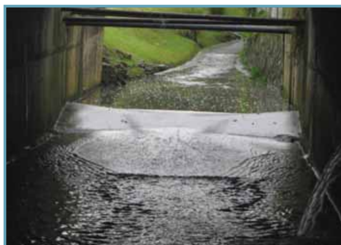
Figure 2 – Eskdale stormwater gauging station – dry weather flow
