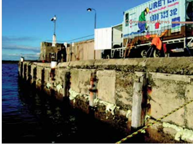
Engineered geo-polymeric structural resins are used to seal seawall
