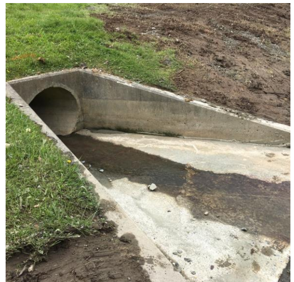
Figure 11: Before & after at main (625 mm diameter) stormwater outfall
