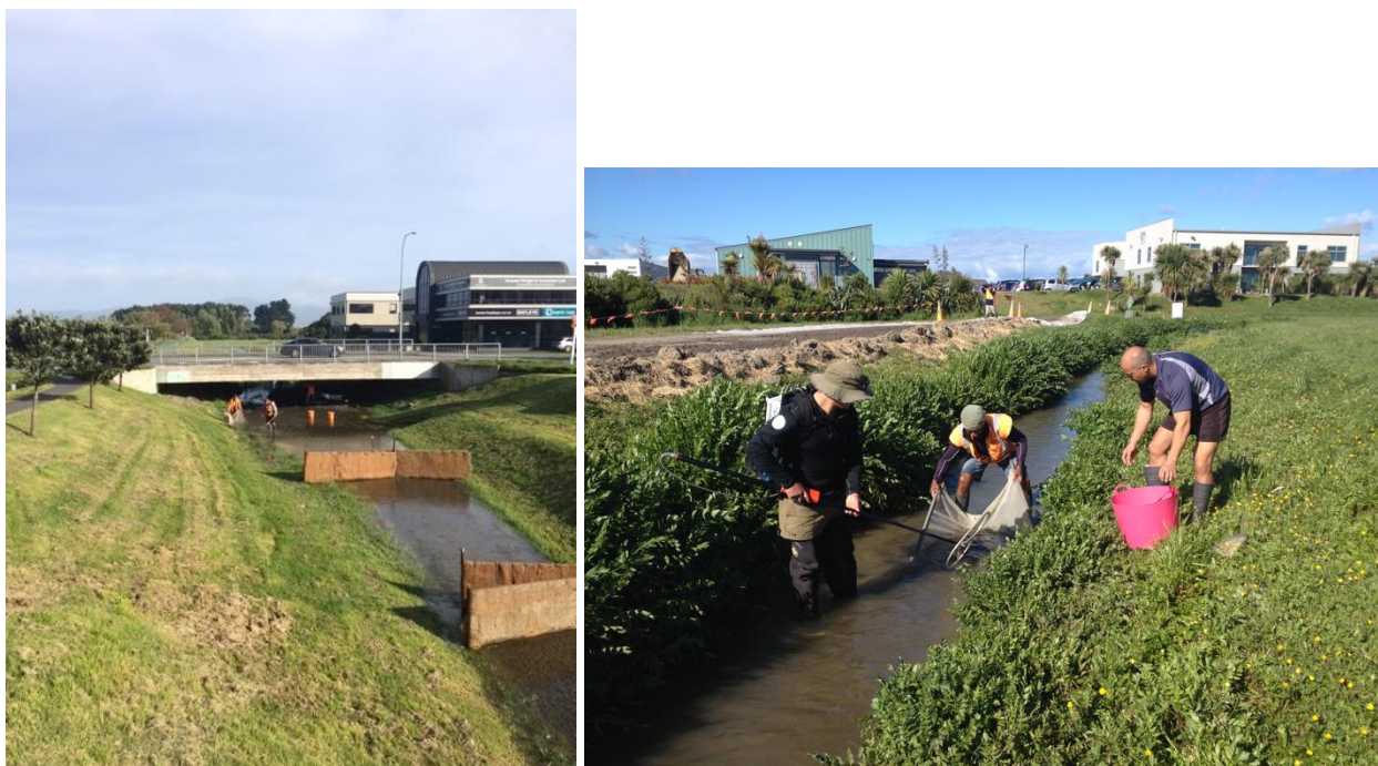
Figure 8: Erosion and sediment control and fish relocation
