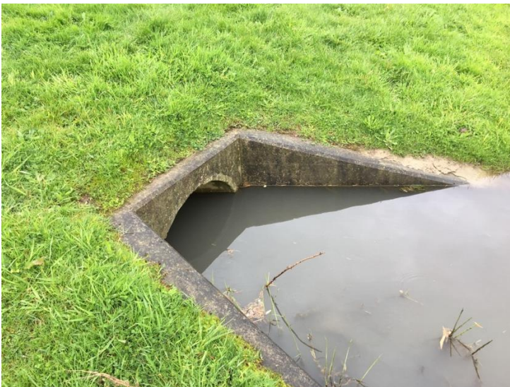
Figure 11: Before & after at main (625 mm diameter) stormwater outfall
