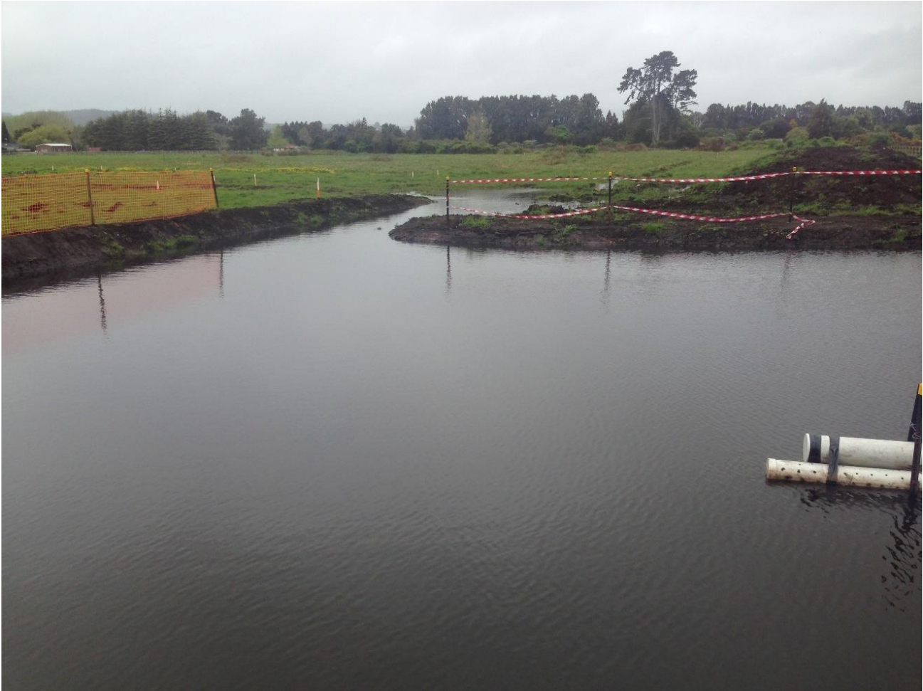
Figure 7 – Temporary Pond sediment retention pond and ground water
