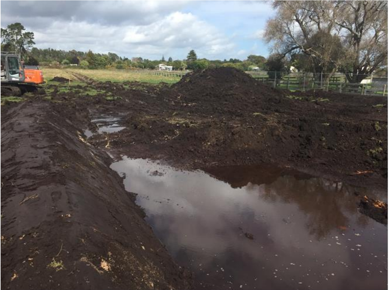
Figure 6 – Condition of peat soils on site
