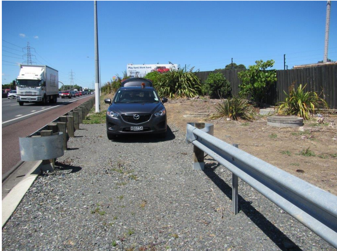
Figure 7: New Guardrail opening. Pre-Sandfilter retrofit (Source: P Mitchell, 2015)
