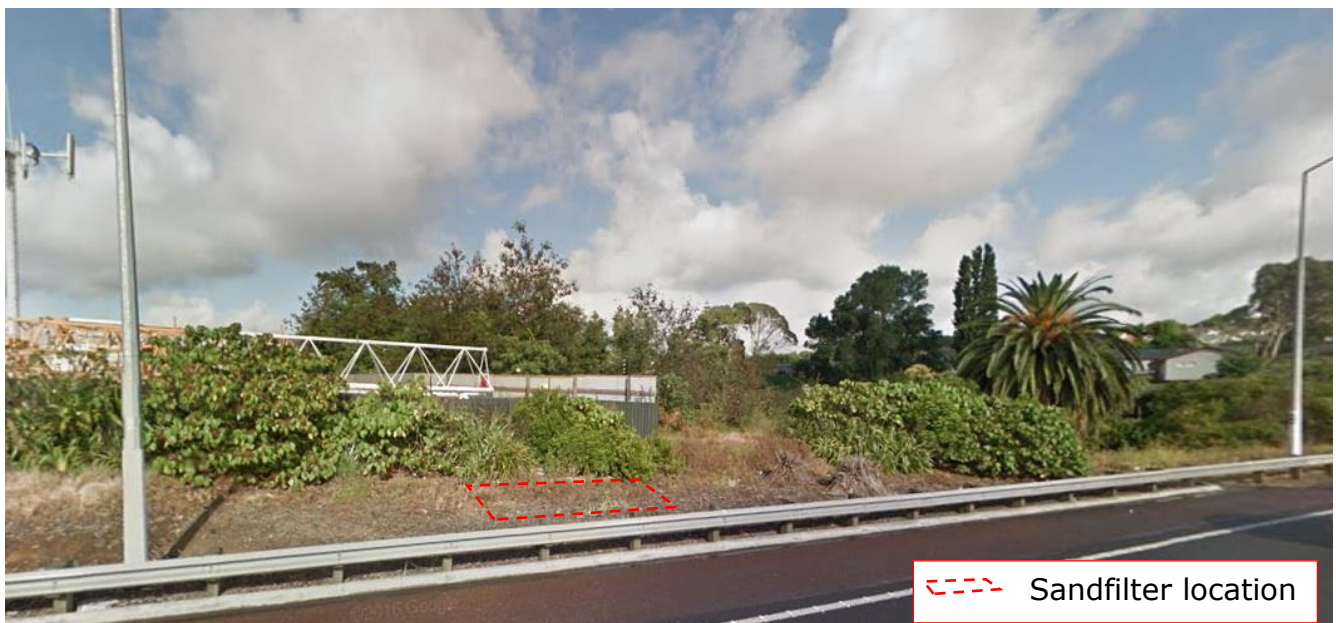
Figure 3: View of Sandfilter site from motorway 2012 (Source: Google)
