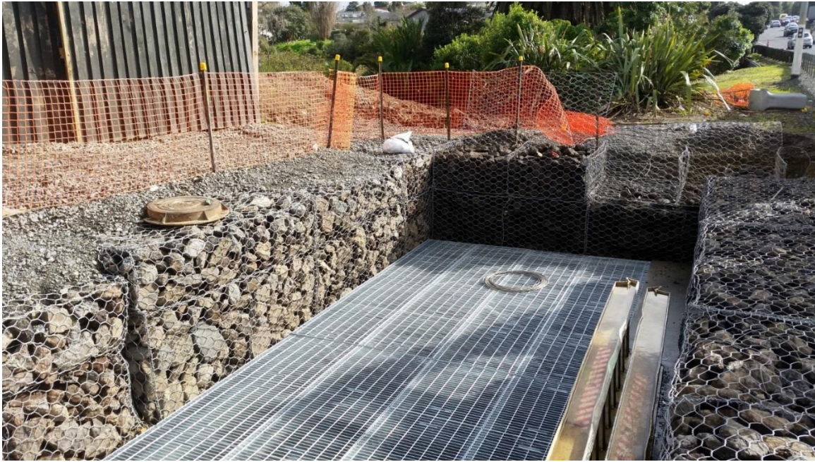
Figure 8: Grated top of StormFilter Retrofit (Source: T Brockbank, 2016)
