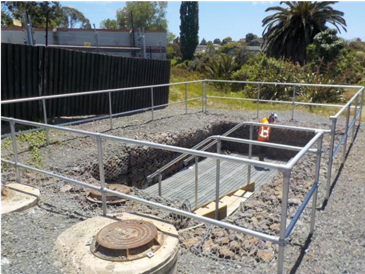
Figure 8: Grated top of StormFilter Retrofit (Source: T Brockbank, 2016)
