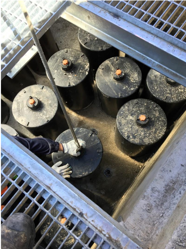
Figure 6: Installing StormFilter Cartridges (Source Stormwater360, 2016)
