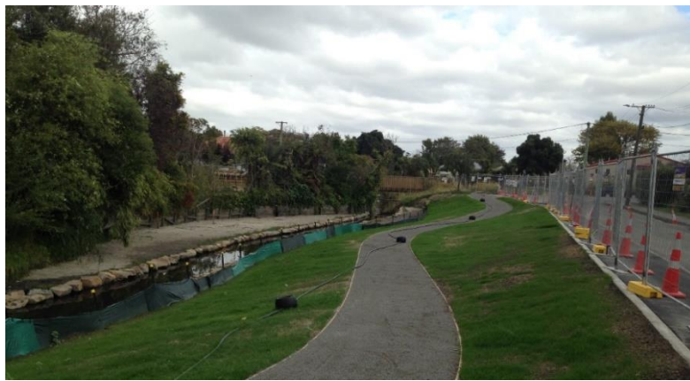
Photograph 10: Realignment of the creek to improve flow
