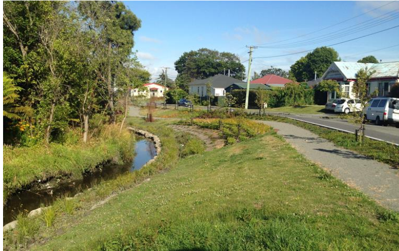
Photograph 10: Realignment of the creek to improve flow
