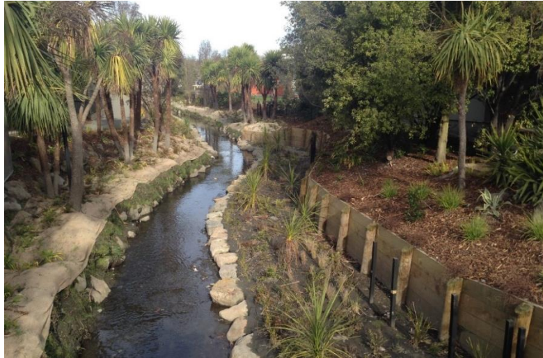
Photograph 7: New retained bank with fresh plain
