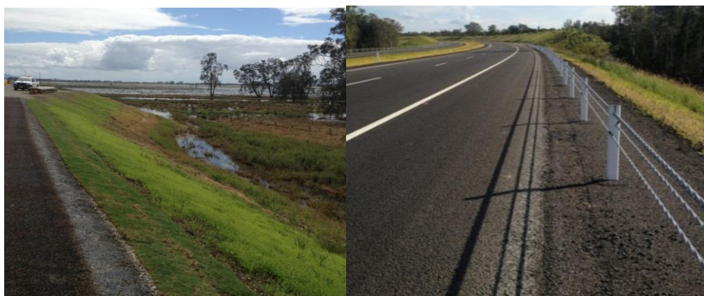
Figure 4 - Highway seal extended over verge and hinge with filter strip and vegetated batter
