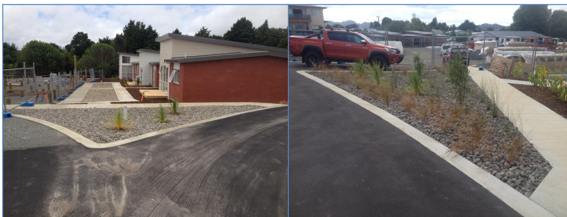
Photograph 1: Flow-through planters at construction and coming on line.
