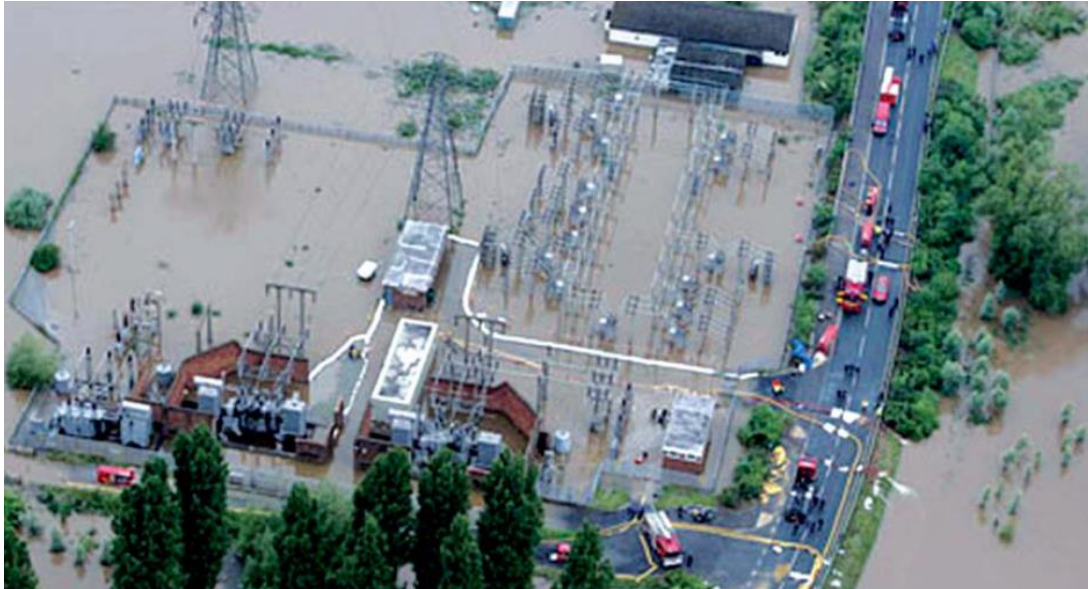
Figure 2 - Castle Meads Electricity Sub-Station flooded during the July 2007 events impacting 40,000 customers for a period of 24 hours
