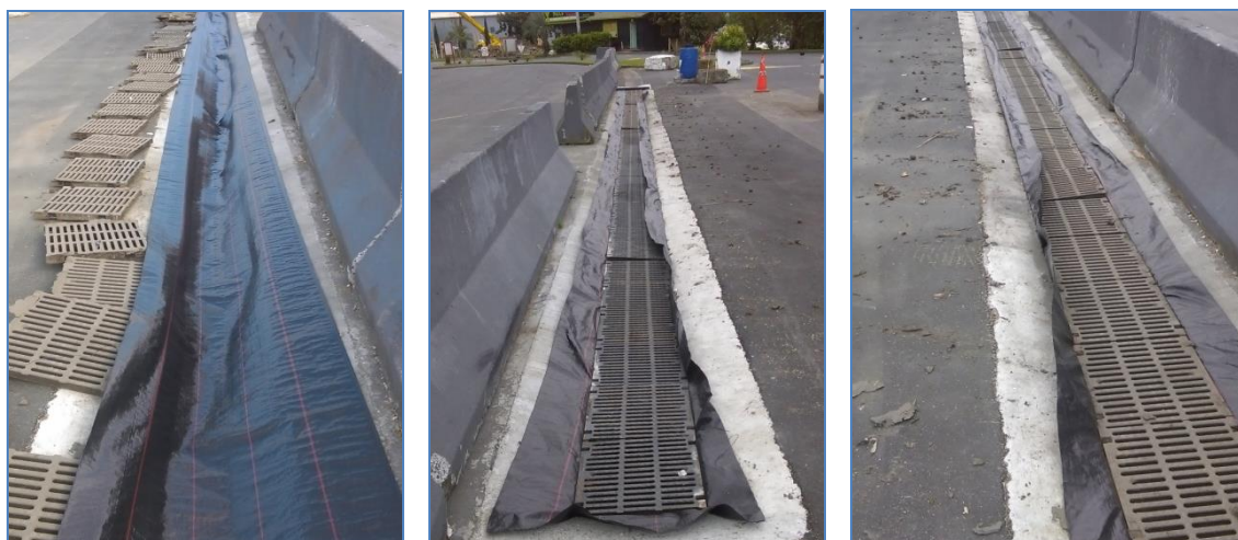
Photograph 3: Addition of filter fabric to treatment drain
