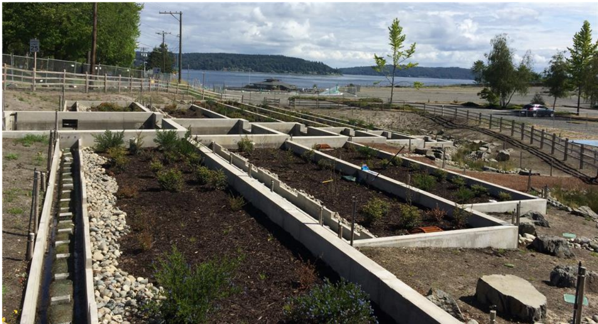
Figure 6: Photo of cascading rapid biofiltration treatment cells at the Point Defiance Stormwater Treatment Facility (Source: Contech Engineered Solutions)
