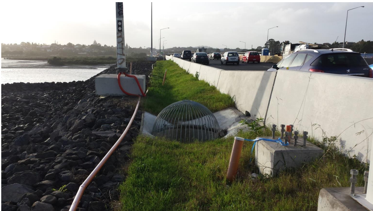
Figure 4: Photo of hybrid Swale & 'scruffy dome' entry Filtration device treatment train (Source: Causeway Alliance)
