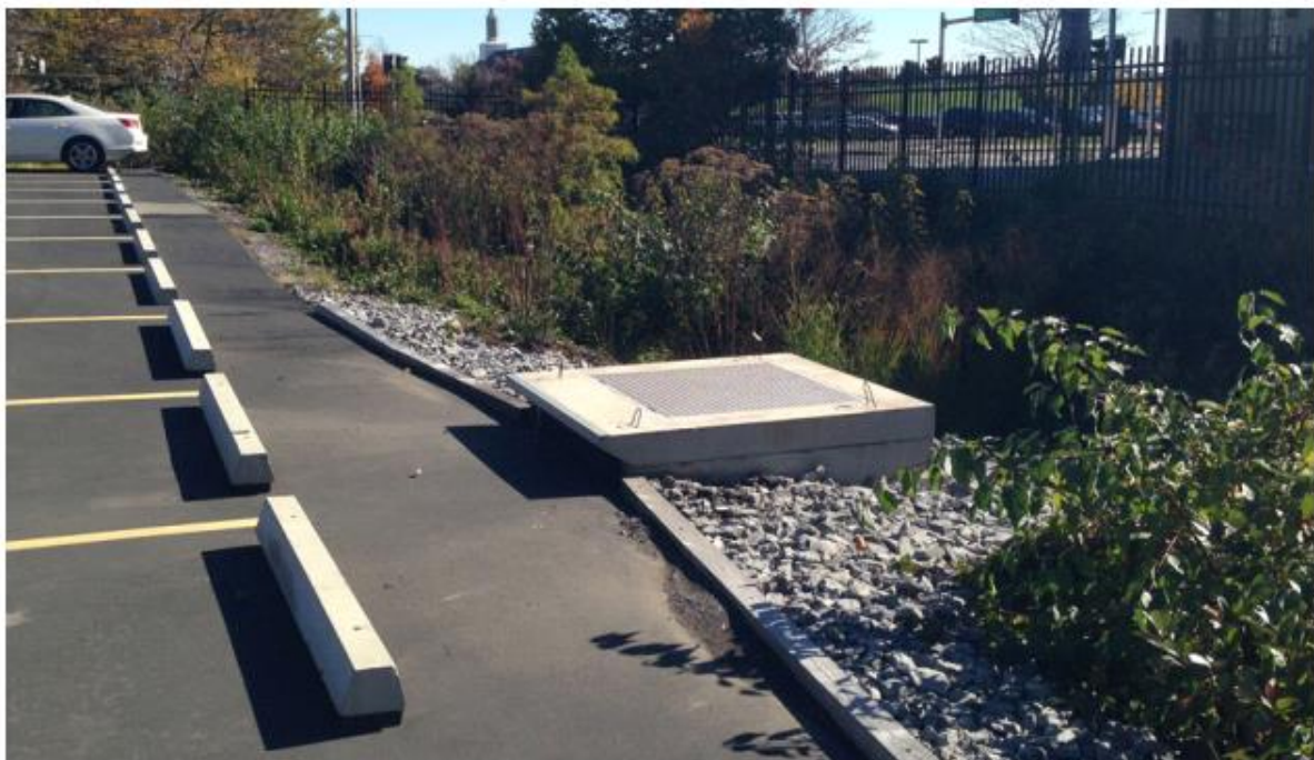
Figure 8: Photo of Hybrid treatment train at Buffalo Niagara Medical Campus (Source: Contech Engineered Solutions)
