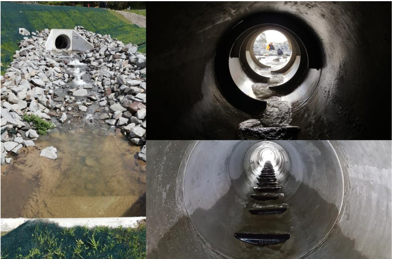
Figure 8: Photographs showing constructed open channel, fish baffles and energy dissipation rings
