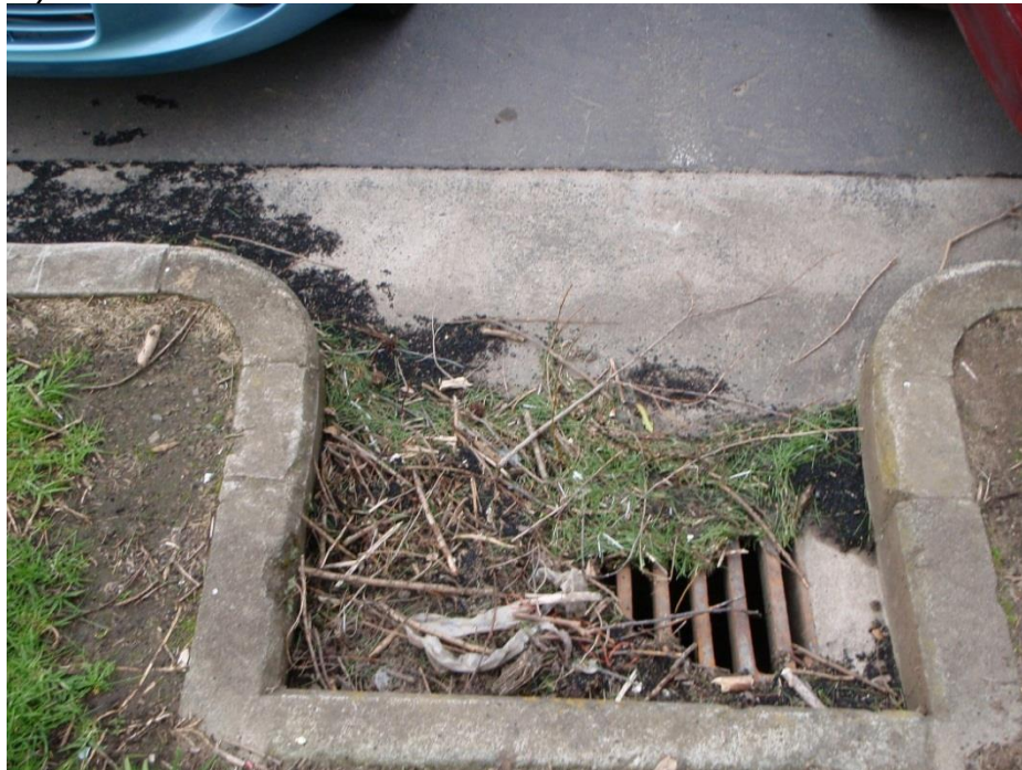
Figure 4: The migration of artificial grass fibres off artificial turf onto nearby hardstanding areas which may then be washed into the local stormwater network
