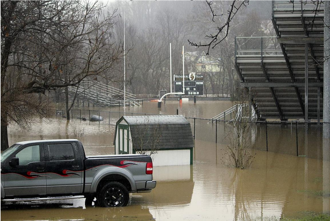
Figure 9: Artificial turf flooding, Waynesburg University, December 2016
