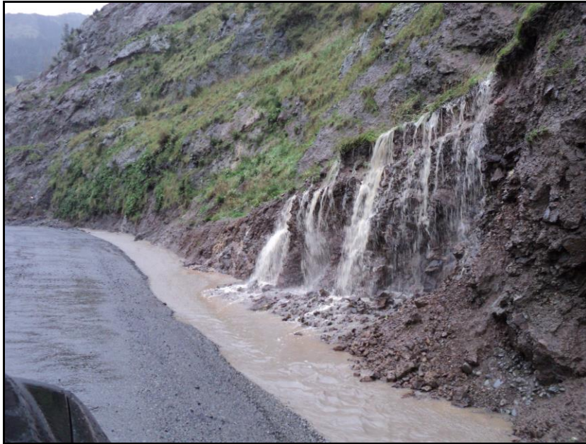
Photograph 1: Flooding adjacent to the existing haul road
