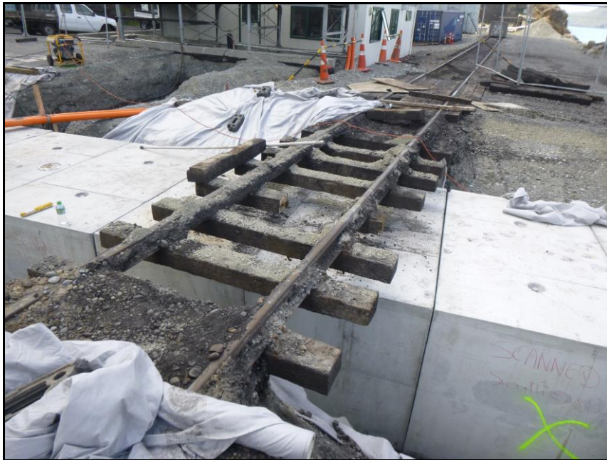
Photograph 3: Box culvert crossing under the existing railway
