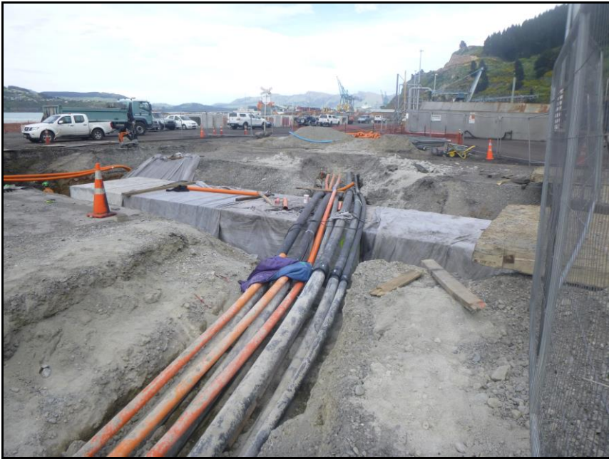
Photograph 4: Re-route of existing services over box culvert
