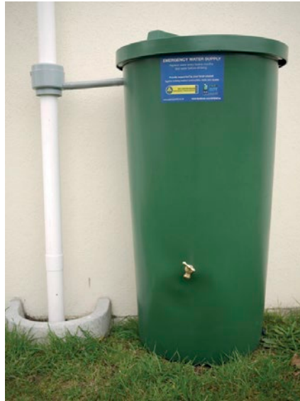
Figure 2: A 200 litre WREMO rain water tank connected to down pipe via water diverter.
