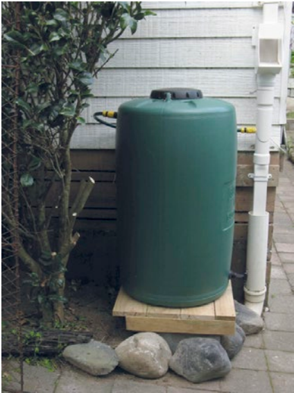
Figure 1: A 250 litre GutterWitch rain water tank connected to down pipe via debris screen and water diverter.
