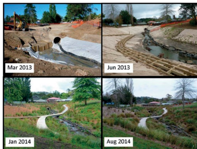
Figure 2: Time series photographs showing the change in channel appearance of the Waitahurangi Stream pre- and post-daylighting.
