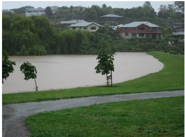
Photographs 1 & 2: Bill Wilkes Detention Basin Outlet (left) Basin full and overflowing at weir (right)
