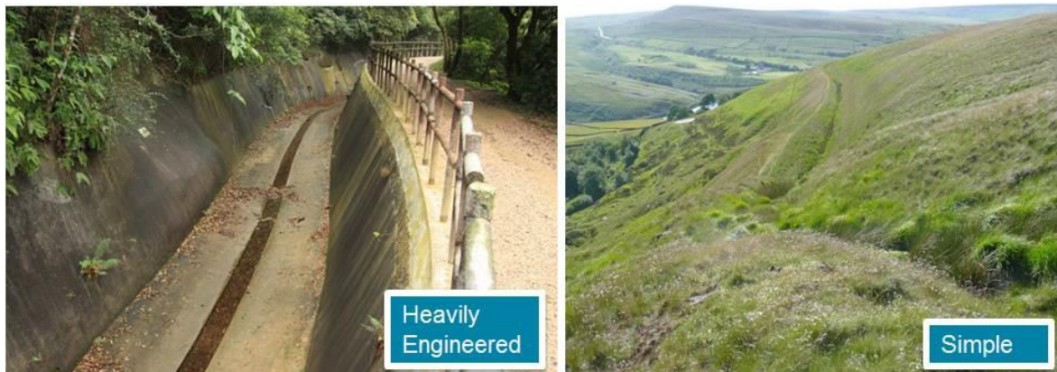
Figure 2: Source control – Catchwater diversion channels
