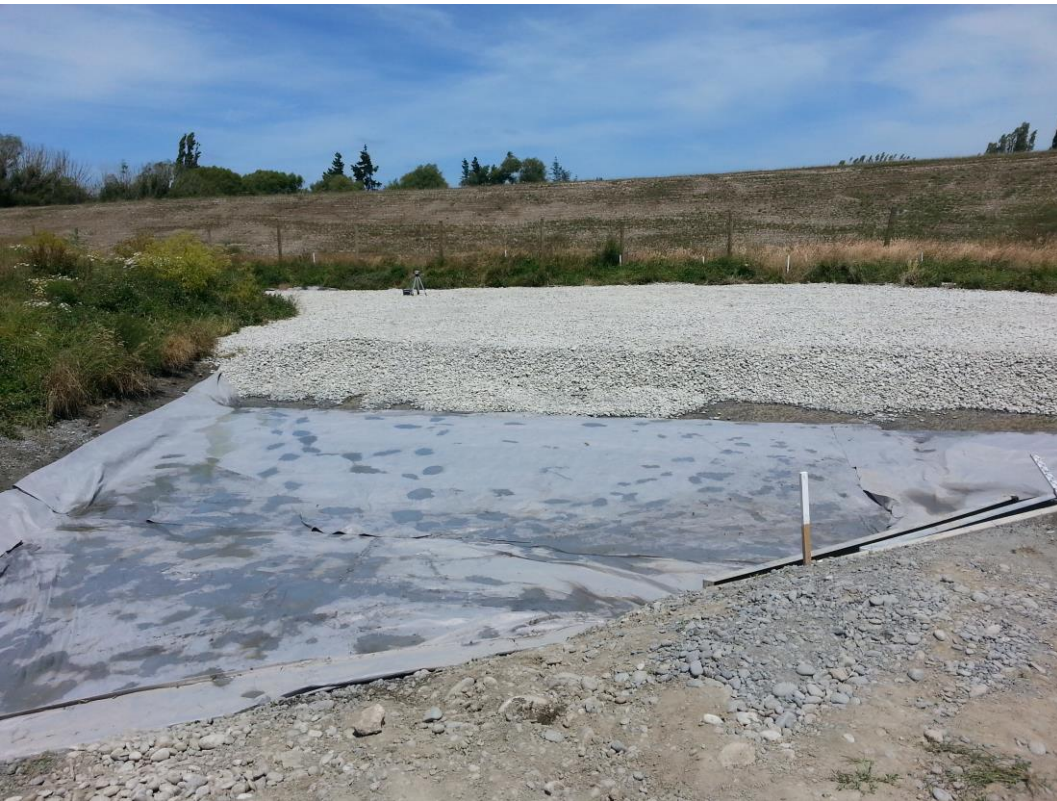
Figure 7 – Placement of the 500mm deep gravel lining underway
