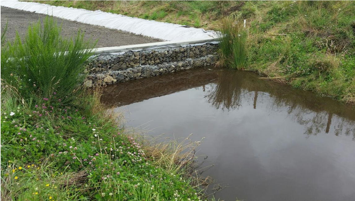
Figure 3 – Sand filter (lined with a sand compost mix), gabion weir wall and wetland forebay pool (post its first rainfall event)
