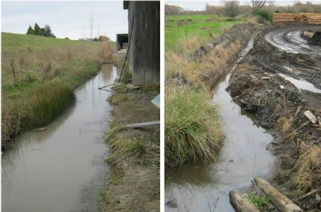
Figure 2 – Ponding water in the perimeter drain prior to the re-development
