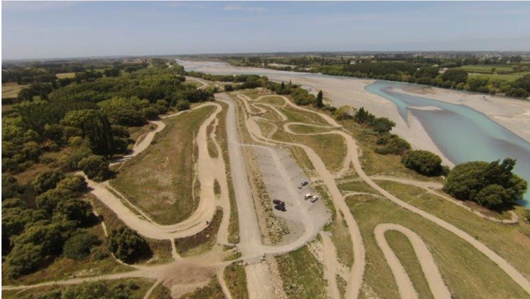
Figure 10: Parking and Bike Track Development in conjunction with Rock Protection Work
