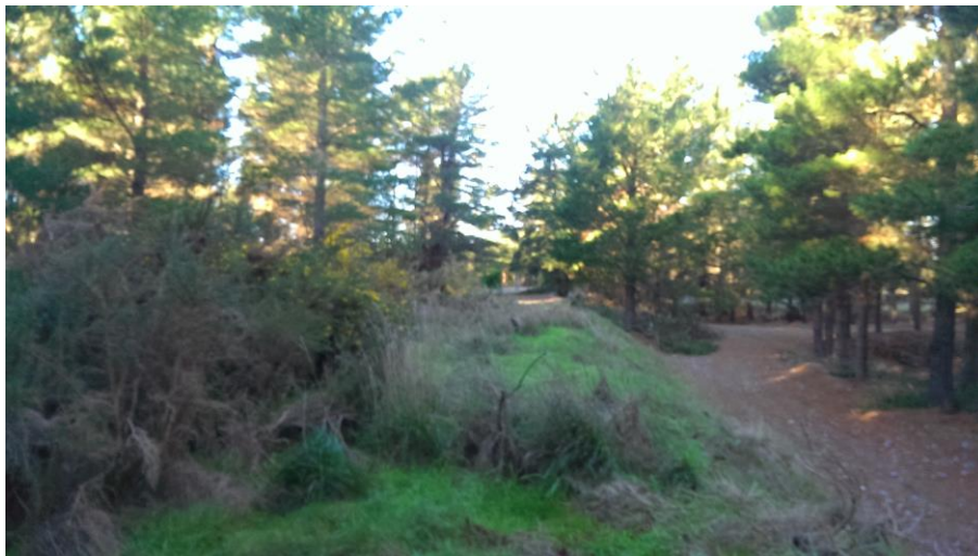
Figure 8: Heavy Vegetation Growth on Historic Stopbank
