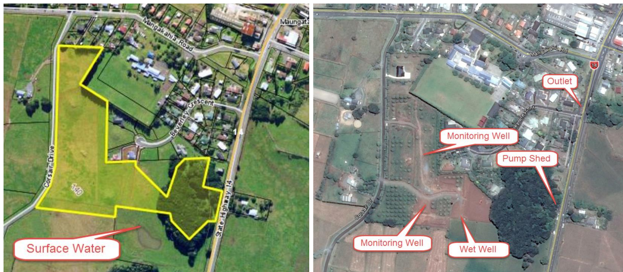
Figure 1: 2002 aerial image showing ponded surface water. A recent satellite image taken during construction
