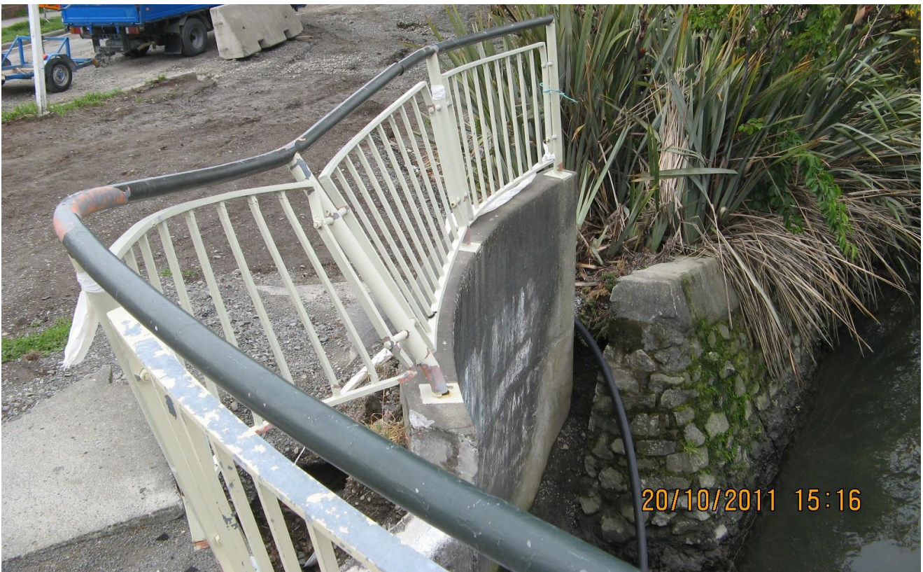
Photograph 3: Example of Direct Damage to Structures (Gayhurst Road Bridge, October 2011)
