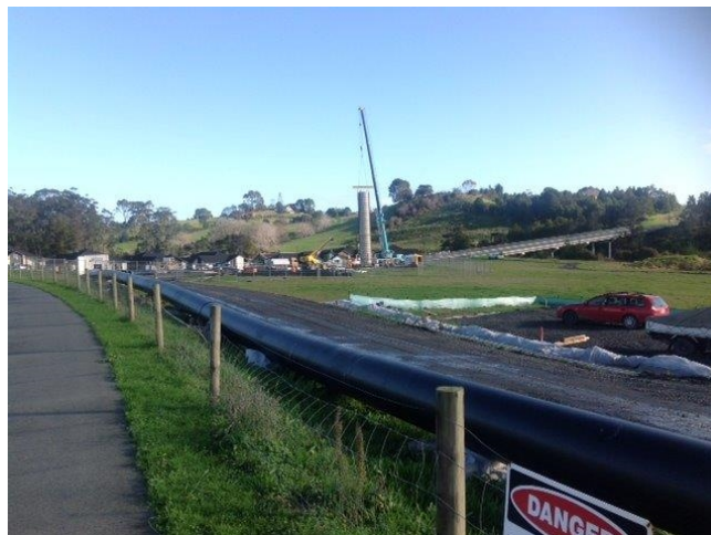
Photograph 2: 600 metre of 630 OD PE pipe string ready to be pulled into place
