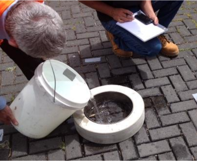
Photo 1: Timing a set volume of water, at a constant depth of 10 to 15mm, to infiltrate the pervious surface within the steel ring. Concrete surround (with a soft closed cell foam on its base, see photos 2 and 3) provides a seal to minimise horizontal leakage from under the inside ring.
