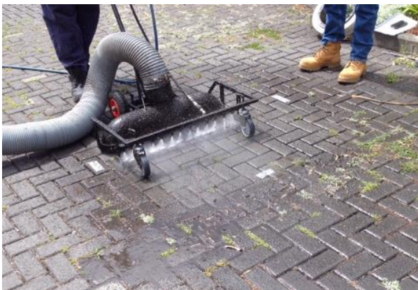
Photos 4 (left) and 5 (right): Cleaning the pervious surface. The thirteen, 1,000 psi water jets dislodge the sediments/moss/weeds from the surface and in the joints, which are then picked up with the vacuum suction. Most weeds are dislodged and vacuumed up but some weeds with long roots remain and need to be hand plucked.
