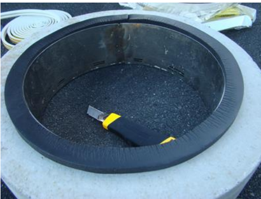
Photo 2: Soft closed cell foam on base of concrete ring.
