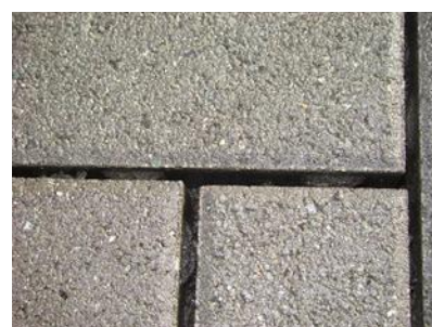
Photo 8: After cleaning, before rechip.
