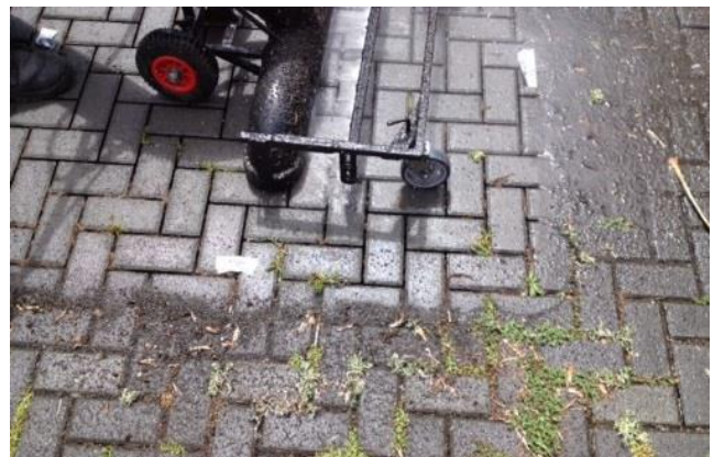
Photos 4 (left) and 5 (right): Cleaning the pervious surface. The thirteen, 1,000 psi water jets dislodge the sediments/moss/weeds from the surface and in the joints, which are then picked up with the vacuum suction. Most weeds are dislodged and vacuumed up but some weeds with long roots remain and need to be hand plucked.
