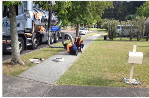
Clemow's Lane, Porous Concrete, Footpath
