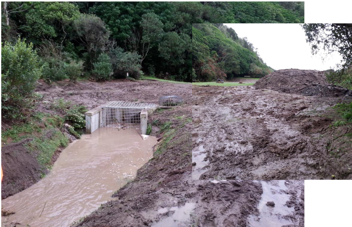
Figure 6 - Inlet structure upstream end of Rangituhi stormwater network
