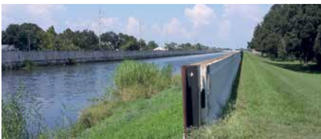
Typical New Orleans levee construction – many failed due to piping and scour under the concrete walls, or over-topping of the walls due to the hydraulic lateral load.
