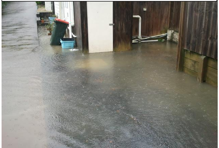
Figure 14: Case Study 6 – combined sewer flooding of private property
