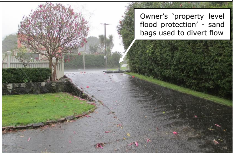
Figure 10: Case Study 4 – reprofiling vehicle crossings so road corridor acts as overland flowpath
