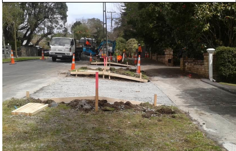
Figure 10: Case Study 4 – reprofiling vehicle crossings so road corridor acts as overland flowpath
