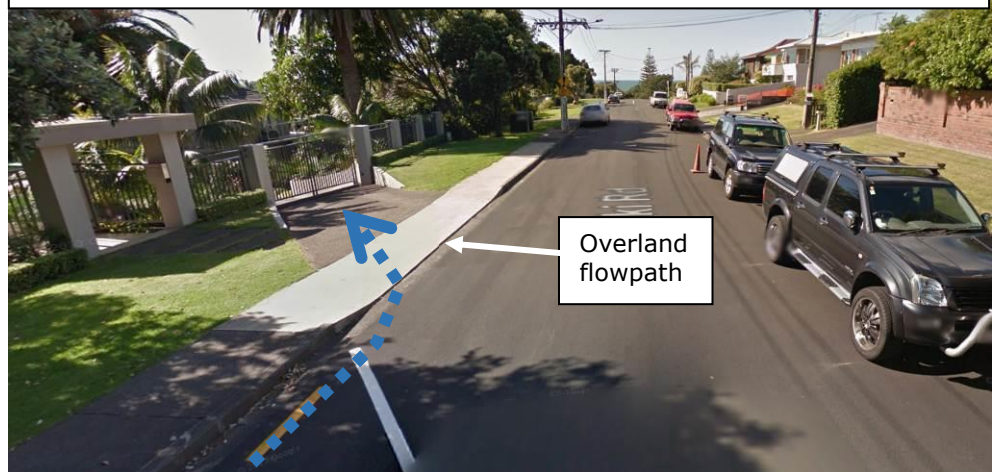
Figure 3: Case Study 1 - overland flow occurs from the road down driveways and into homes
