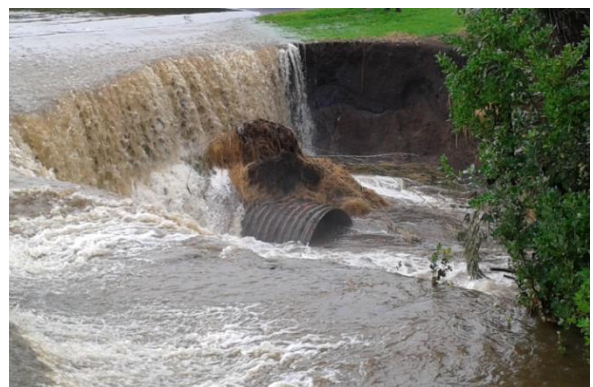
Figures 10 and 11 - Dieffenbach Culvert Failure
