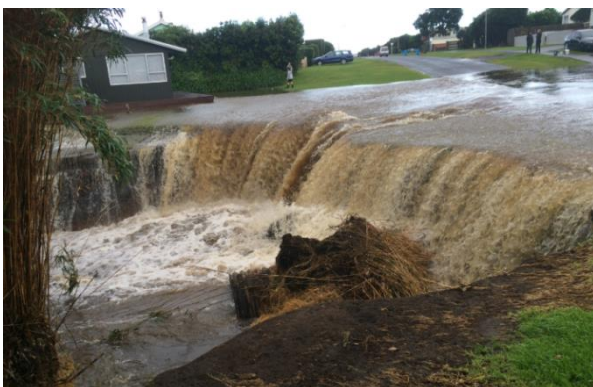
Figures 10 and 11 - Dieffenbach Culvert Failure
