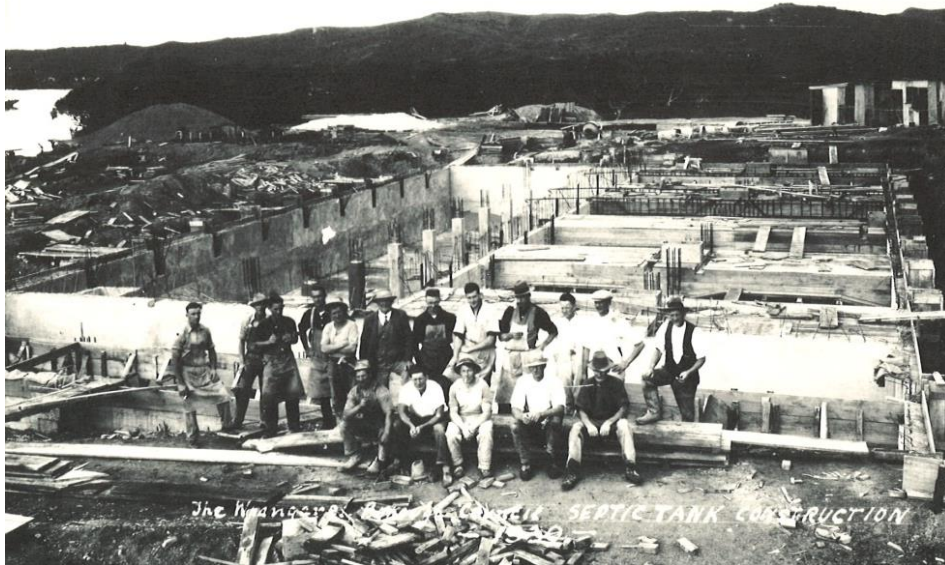
Figure 1: Construction of the Whangarei Septic Tank (1930)
