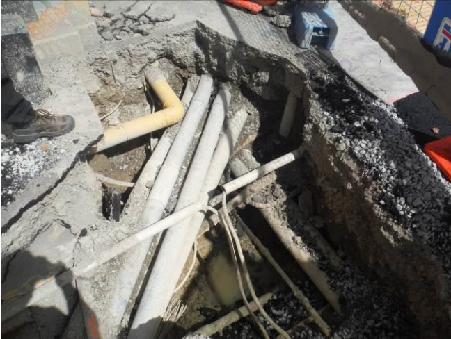
Photograph 1: Existing Services at the Intersection of Victoria Street and Vivian Street
