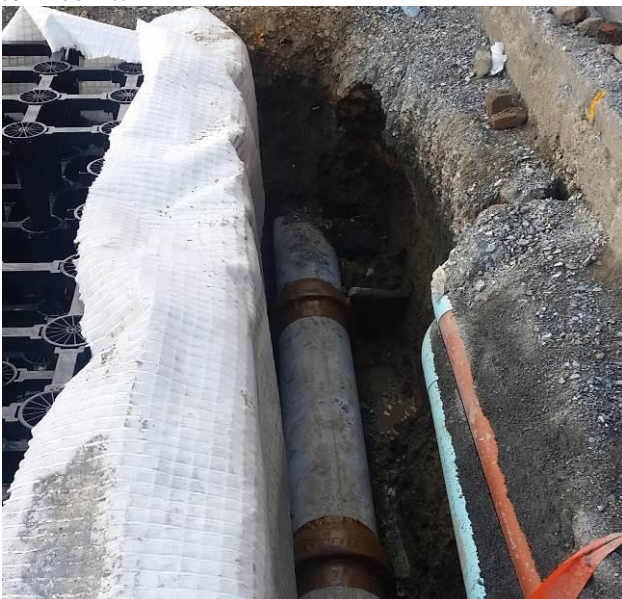
Photograph 3: Densotape of Pipe Joints Adjacent to Tree Pit
