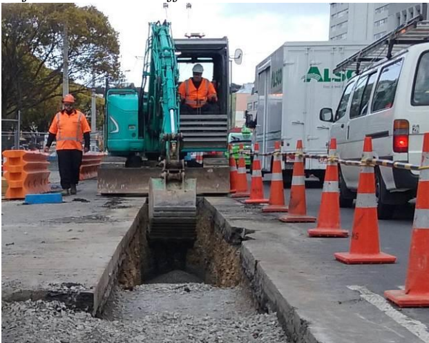
Photograph 5: Trenching Beneath Carriageway Adjacent to Live Traffic
