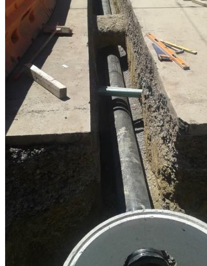
Photograph 2: Installation of Stormwater Pipe Below Existing Services
