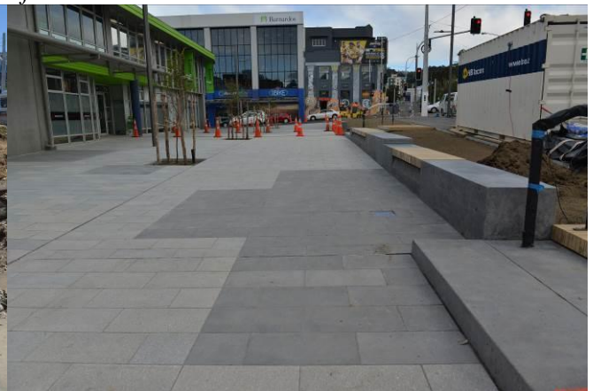
Photograph 8: Geometry of Pocket Park Location After Construction with Central Slot Drain
