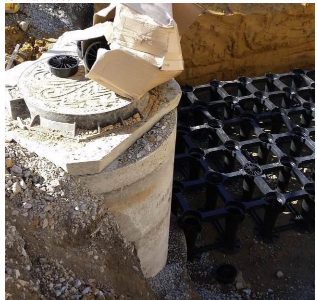
Photograph 4: Construction of Tree Pit Adjacent to Manhole
