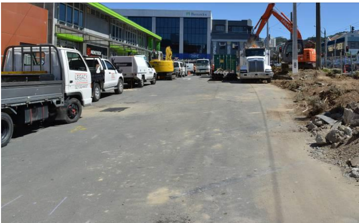
Photograph 7: Geometry of Pocket Park Location Prior to Construction
