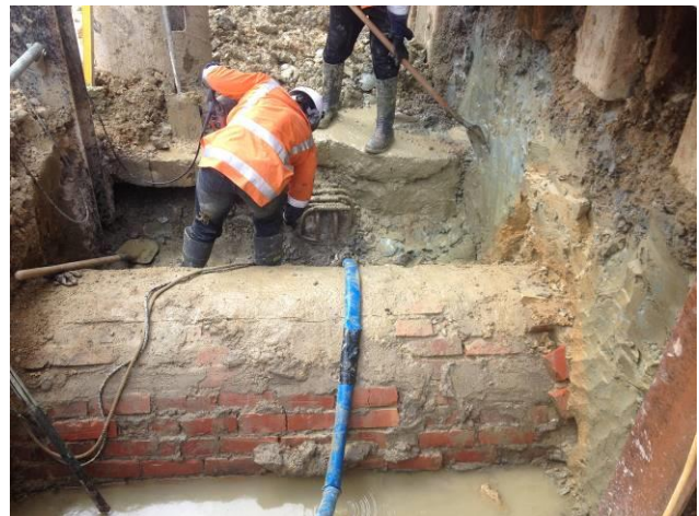
Photograph 3: Tory Street Historical Sewer Exposed
