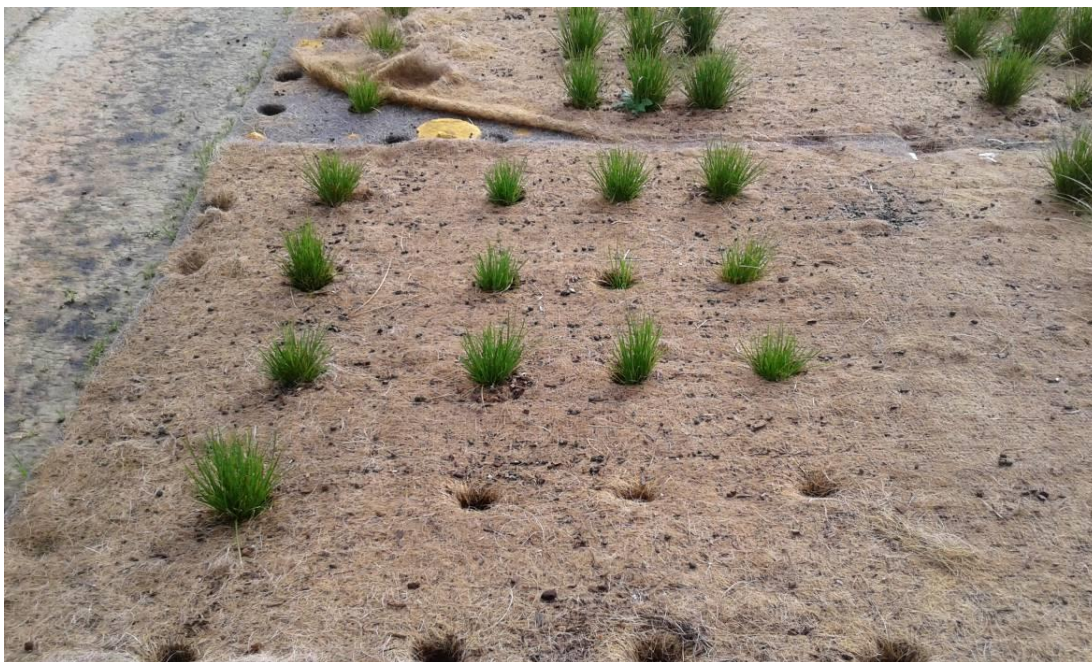
Photograph 9: Close-up photograph of the plants displaying stunted growth (including losses) on the FTM wetlands at Waipu WWTP.
