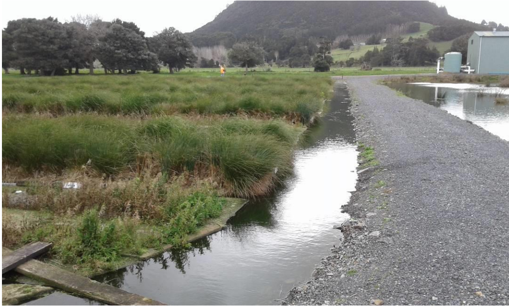
Photograph 6: Photograph of the established FTM wetland at Hikurangi WWTP.
