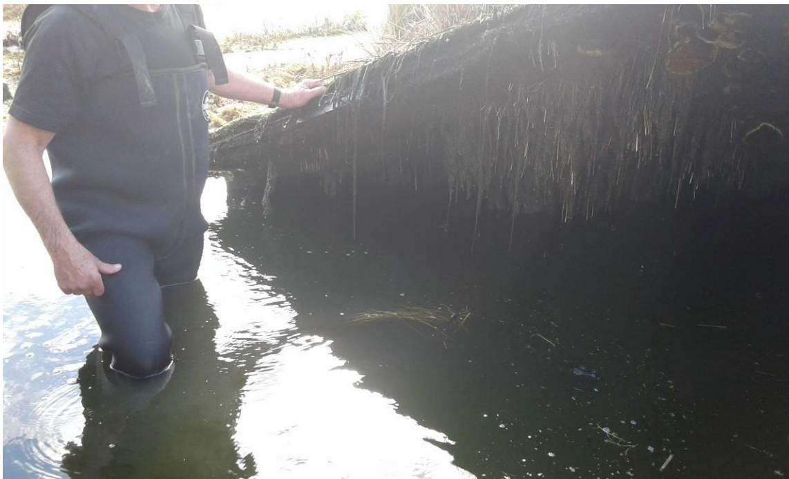
Photograph 7: Lifting of one of the floating pods on the Hikurangi WWTP wetland.
