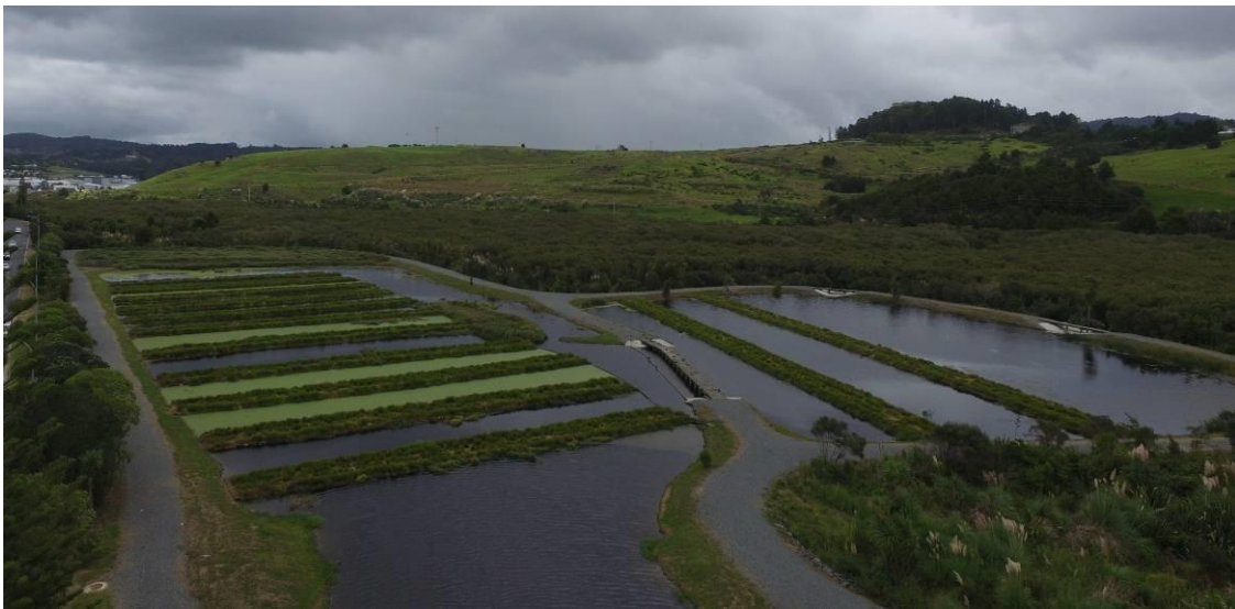
Photograph 1: Floating wetland systems installed at Kioreroa Road WWTP
