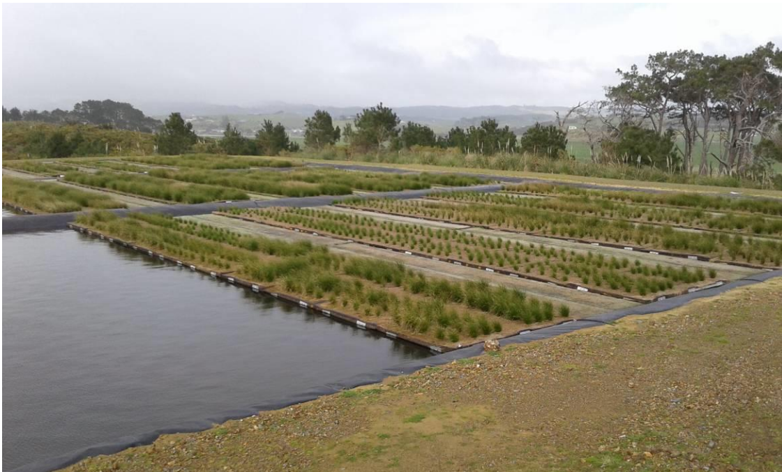
Photograph 8: Overview photograph of the floating wetlands at Waipu WWTP.
