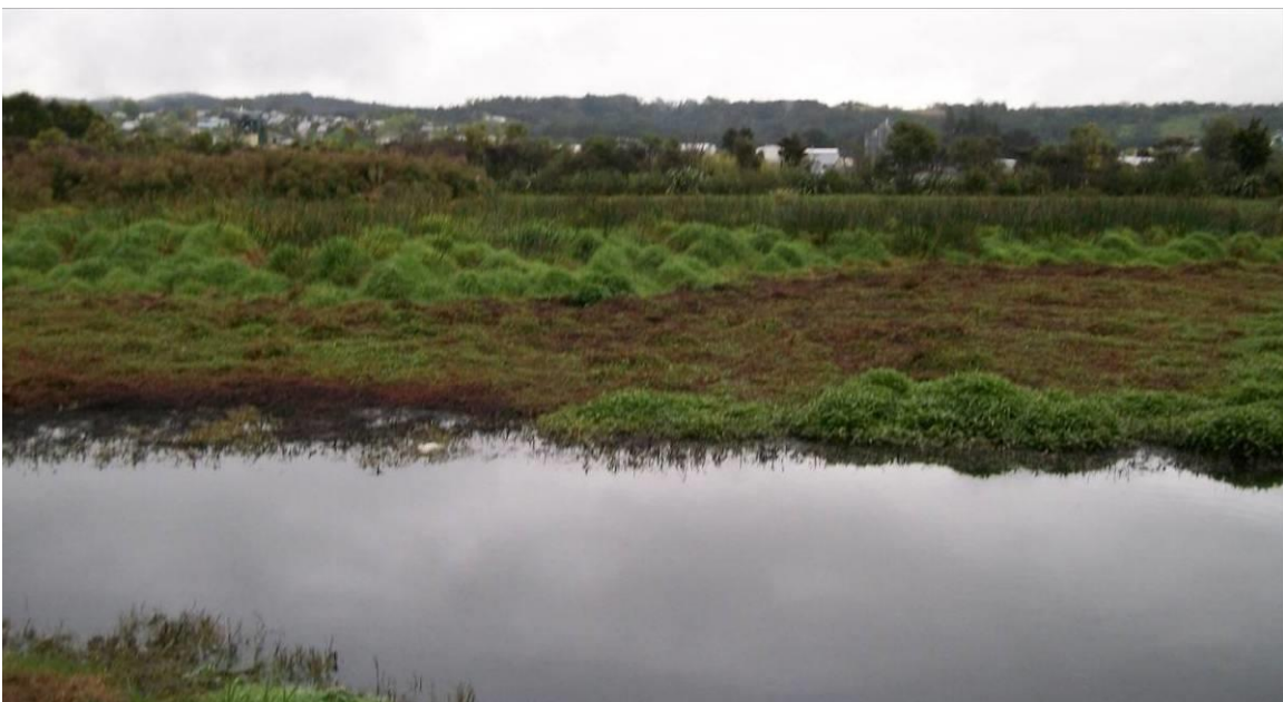
Photograph 2: Kioreroa Road WWTP Wetland Sept 2013 prior to de-sludge and FTM system installation
