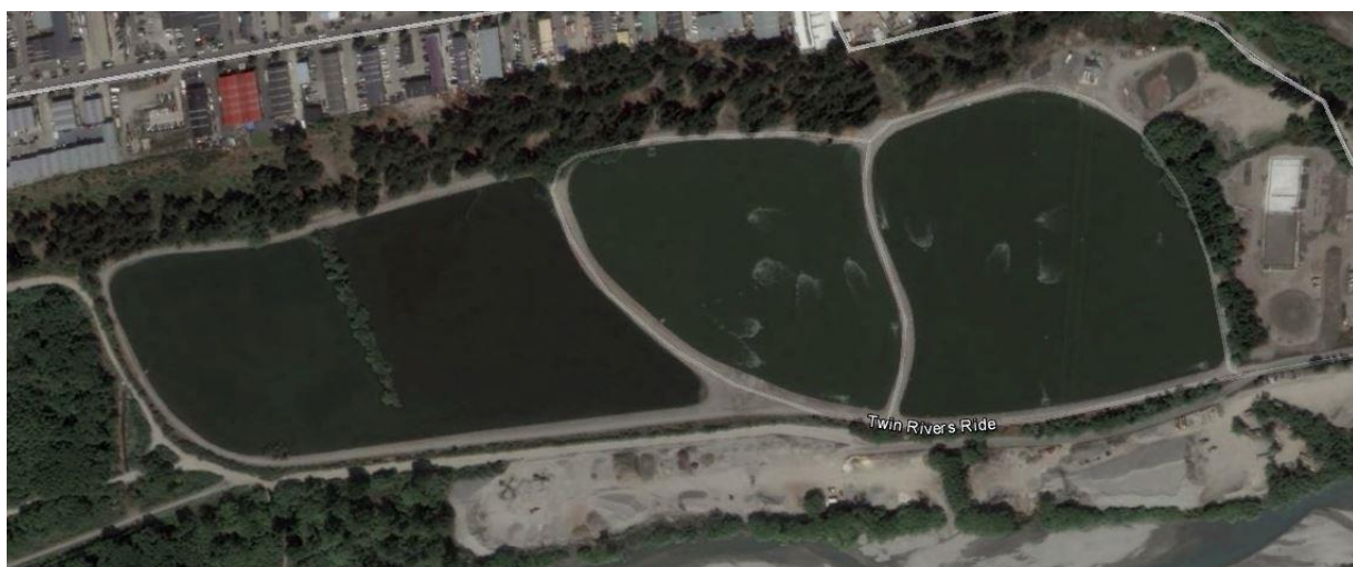
Photo 3: Shotover oxidation ponds at Queenstown
