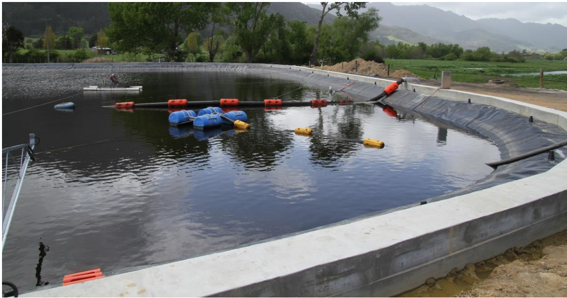
Photograph 6: Completed Relined SBR in Normal Operation
