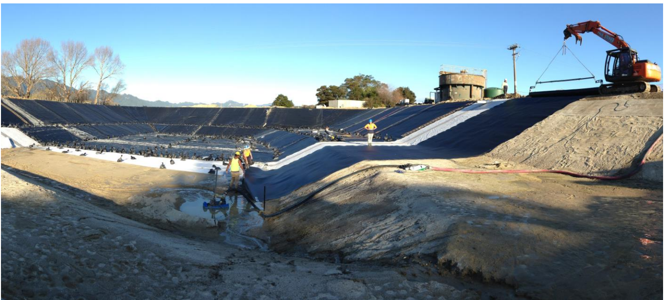
Photograph 5: Relining of the SBR underway
