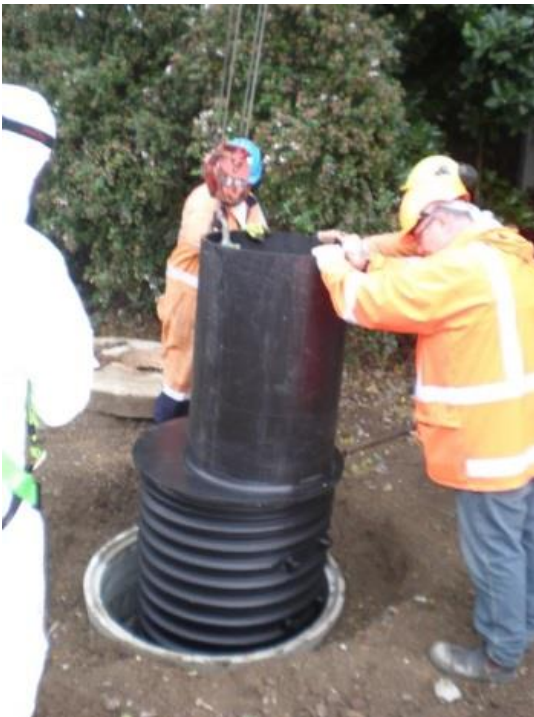
Photo 5: PE Plastic Manhole Inserted into the Existing Corroded Concrete Manhole.
