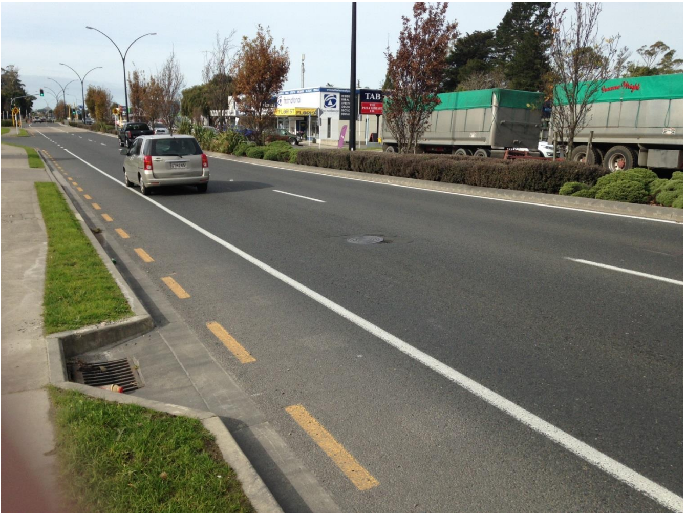
Photo 3: Difficult Access to Trunk Main Manholes in SH2 Bethlehem.
