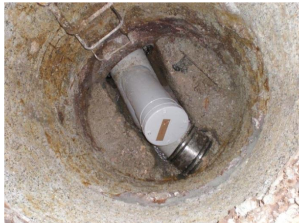
Photo 6: UPVC Plastic Pipe Insert across the Existing Concrete Manhole.
