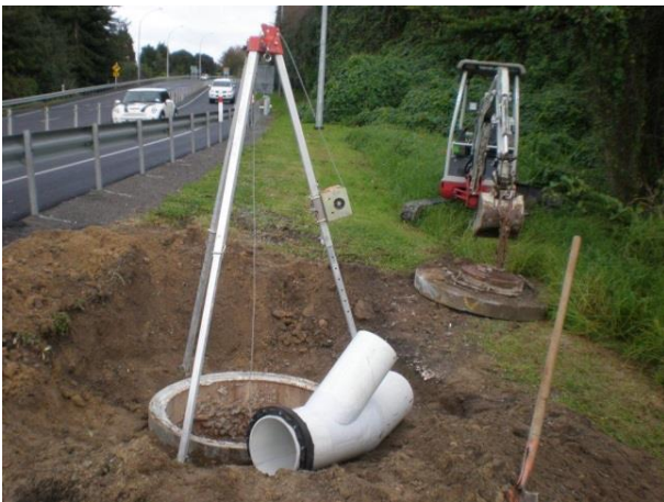
Photo 6: UPVC Plastic Pipe Insert across the Existing Concrete Manhole.
