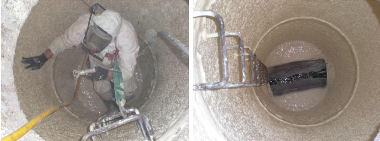
Photo 7: Apply a High Grade Epoxy Coating to the existing Concrete Manhole
