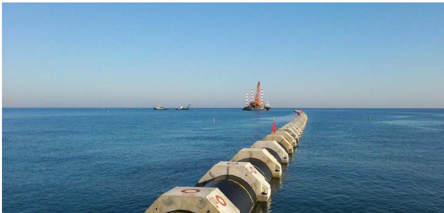
Photo 5 - Pipe is positioned and ready for start of submerging
