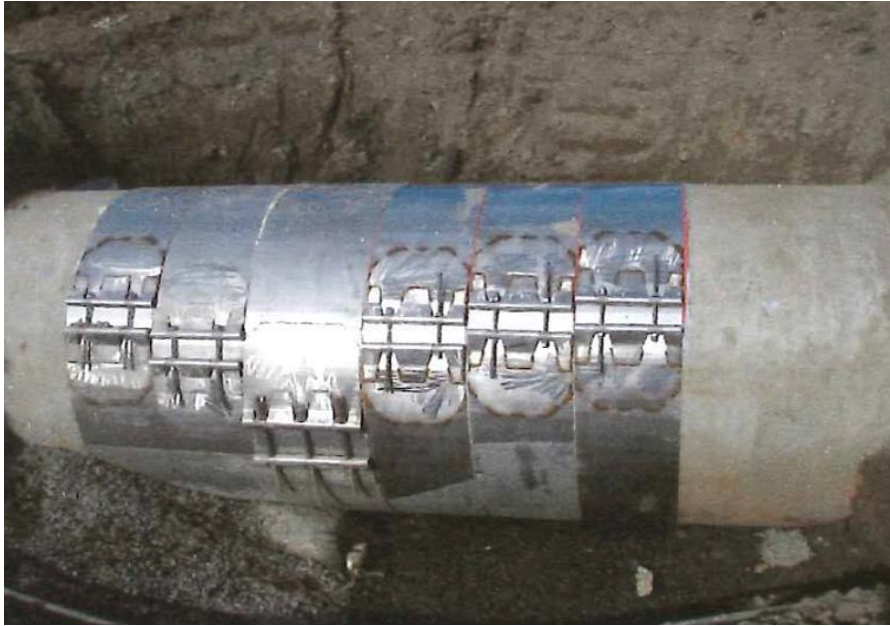
Photograph 2: Concrete Pipe Repair Bands
