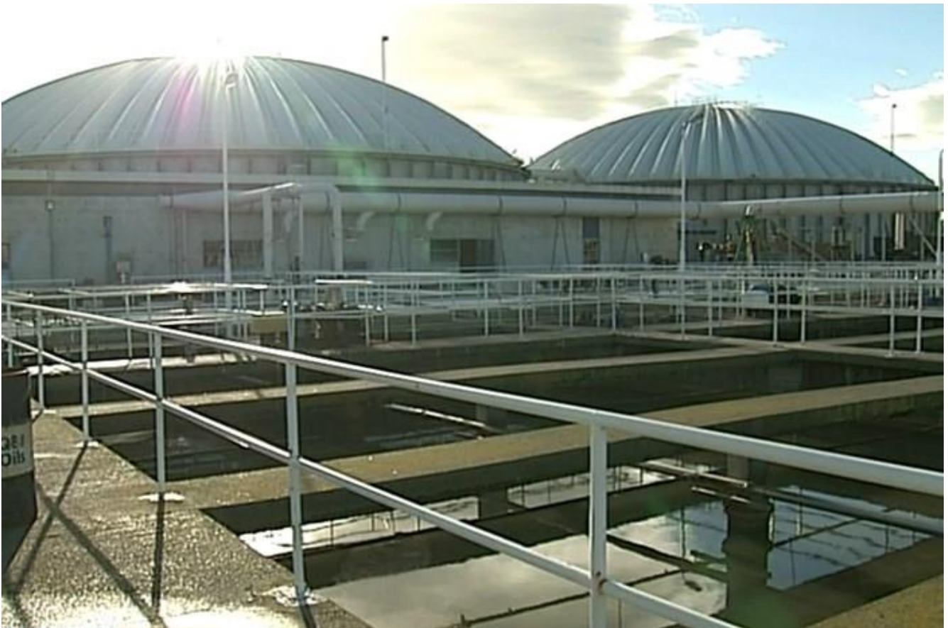
Figure 2: CWTP Trickling Filters
