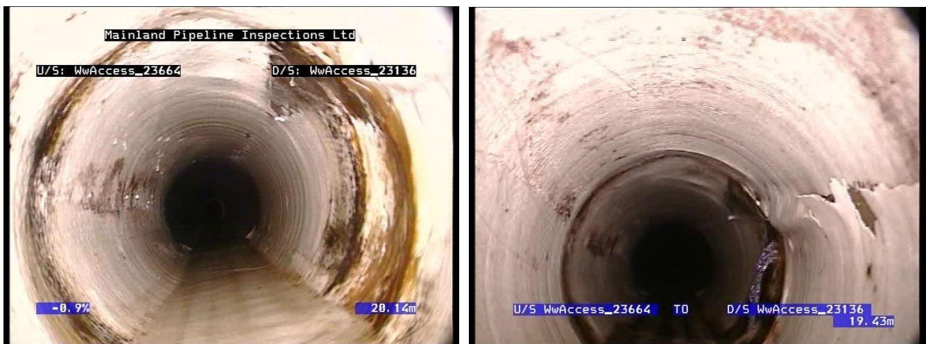
Figure 5 – 2015 CCTV Survey (left), 2016 CCTV Survey (right)
