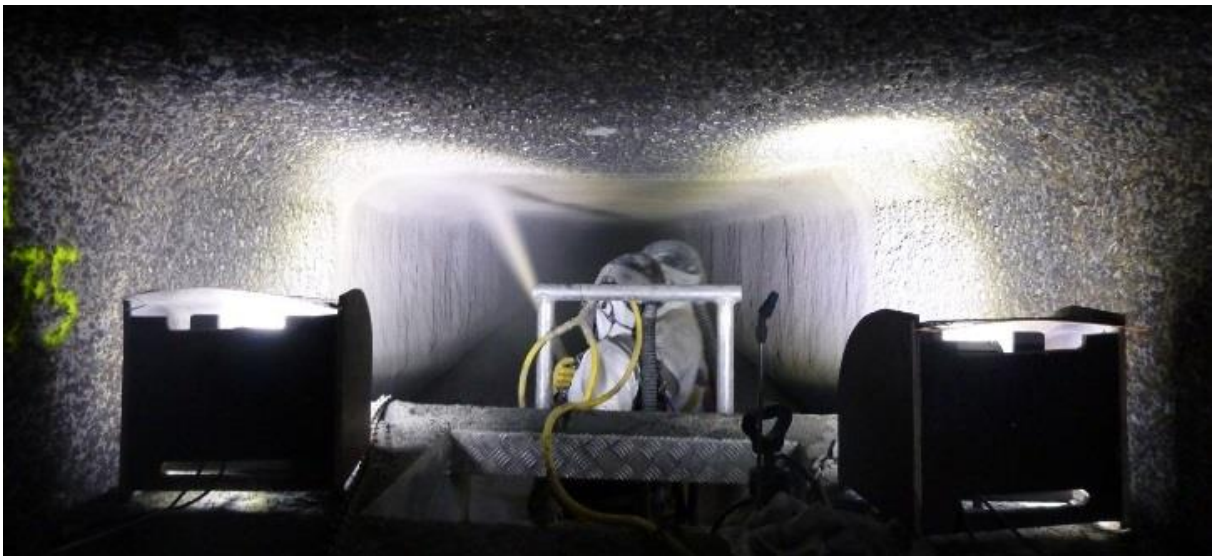
Figure 5. Application of SewperCoat® at the WWTP (SP1)
