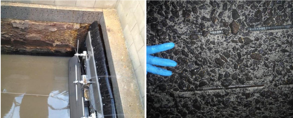
Figure 4 Hydro-demolition cleaning trolley (left), and post substrate clean/preparation (right)
