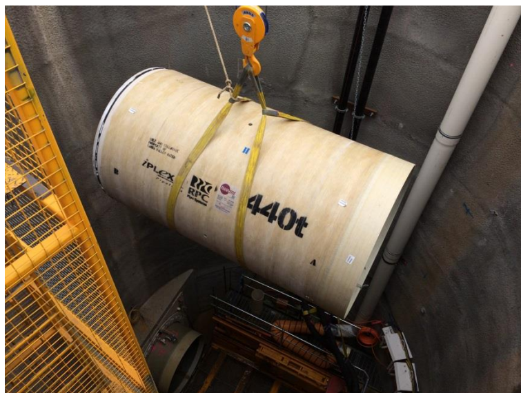
Photograph 5: Amaroo Sewer Main project
