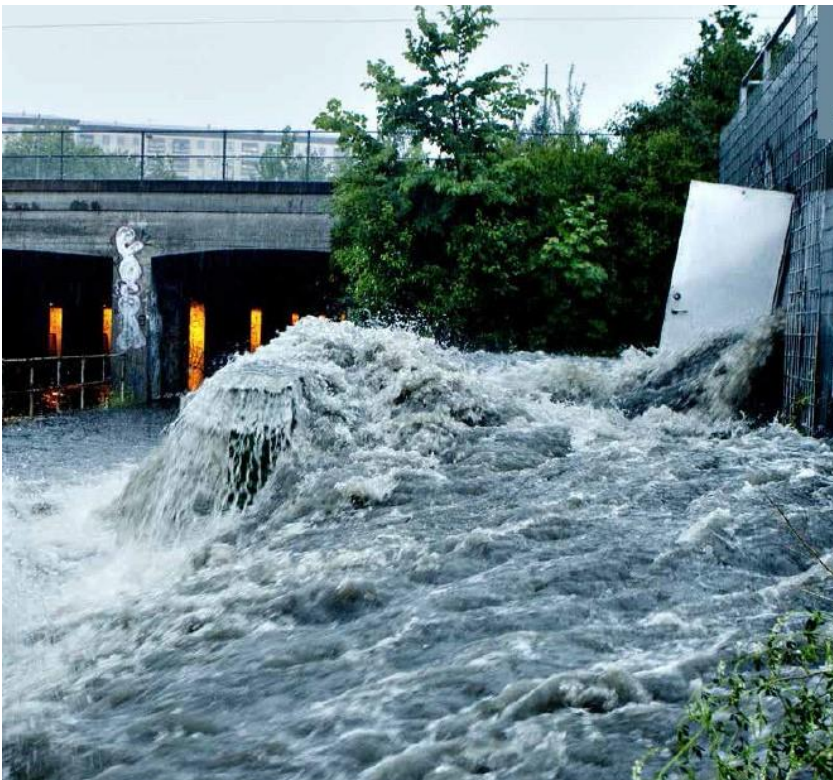
Figure 10: Hazardous impacts of Copenhagen's cloudburst event in 2011 (City of Copenhagen, 2012).
