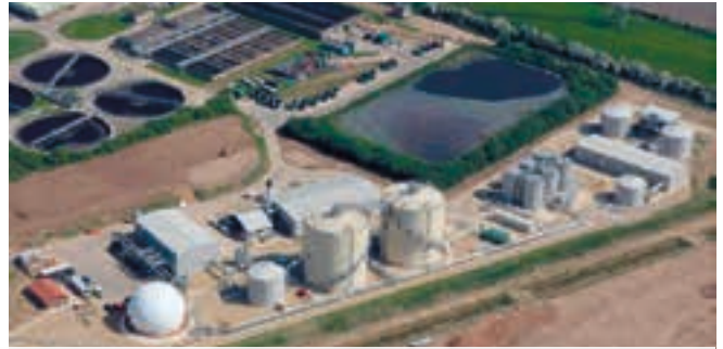
King’s Lynn Biosolids Treatment Centre (foreground) uses biogas CHP to generate sufficient power for the entire wastewater treatment plant.
