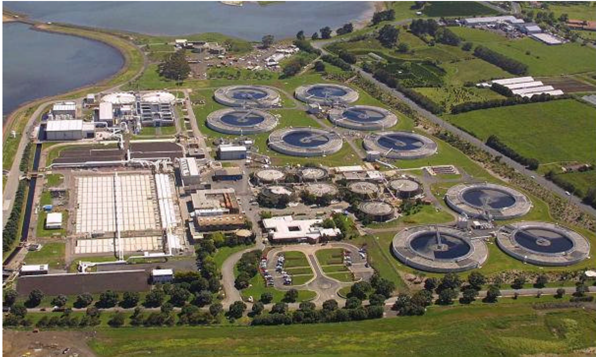
Figure 1: Aerial View of the Mangere WWTP
