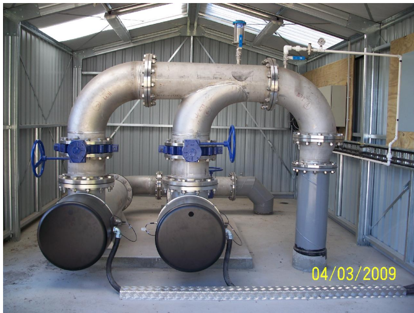
Figure 4. Rotorua Eastern Water Supply's UV Reactors Installation
