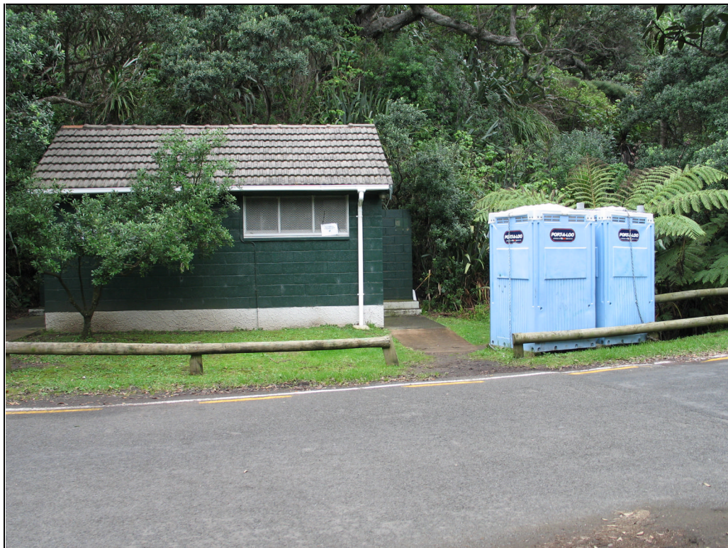
Photograph 1: Karekare Public Toilets – Now Decommissioned
