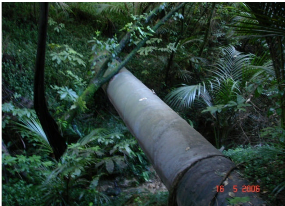
Photograph 1: Typical Terrain around the Horizontal Sections of the Inverted Siphons
