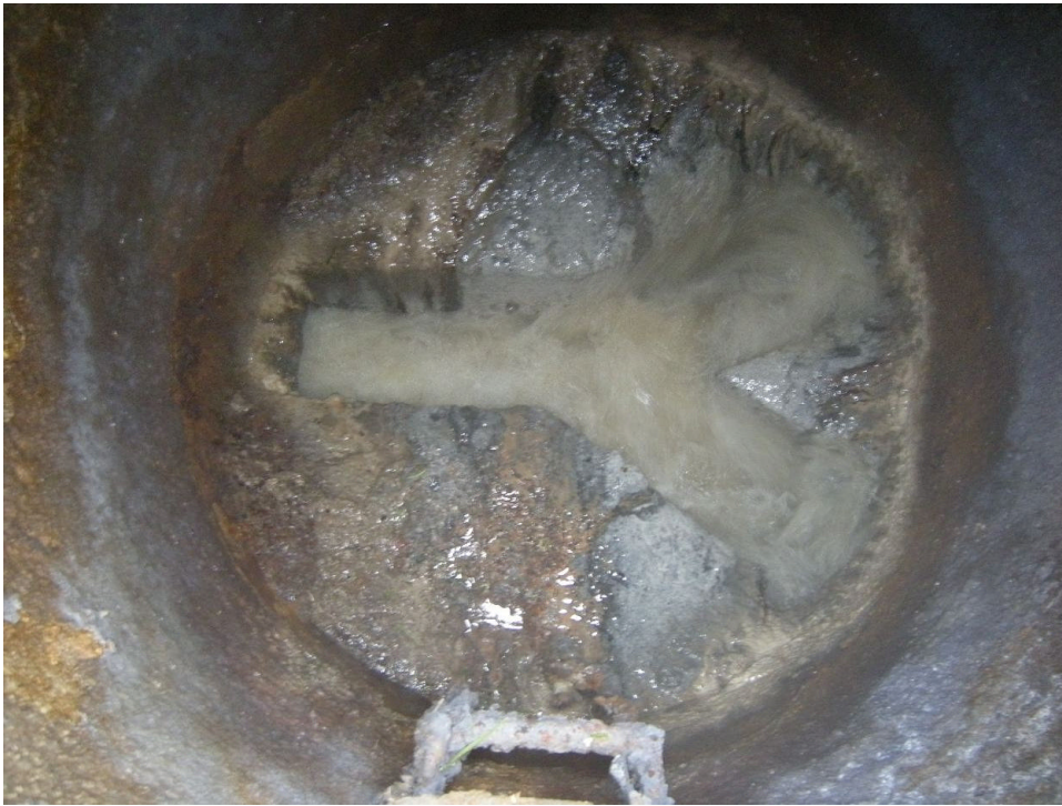
Photograph 8: Behaviour at 70 l/s after installation of air release
