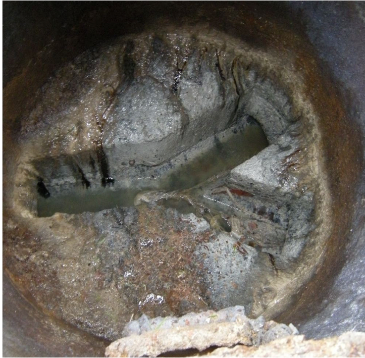
Photograph 6: Siphon Inlet Layout - Flow from left to right
