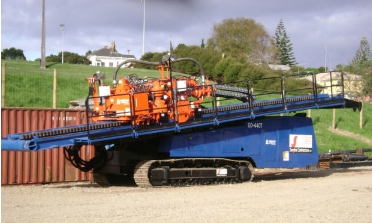
Photograph 5: DD 440T delivered to site (Courtesy of Smythe Contractors)
