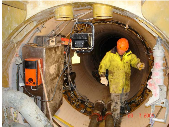
Figure 5-3: trenchless technologies are often used
