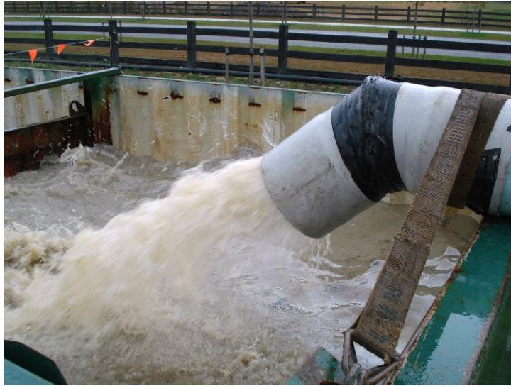
Figure 3. Well development by excessive air lift pumping.
