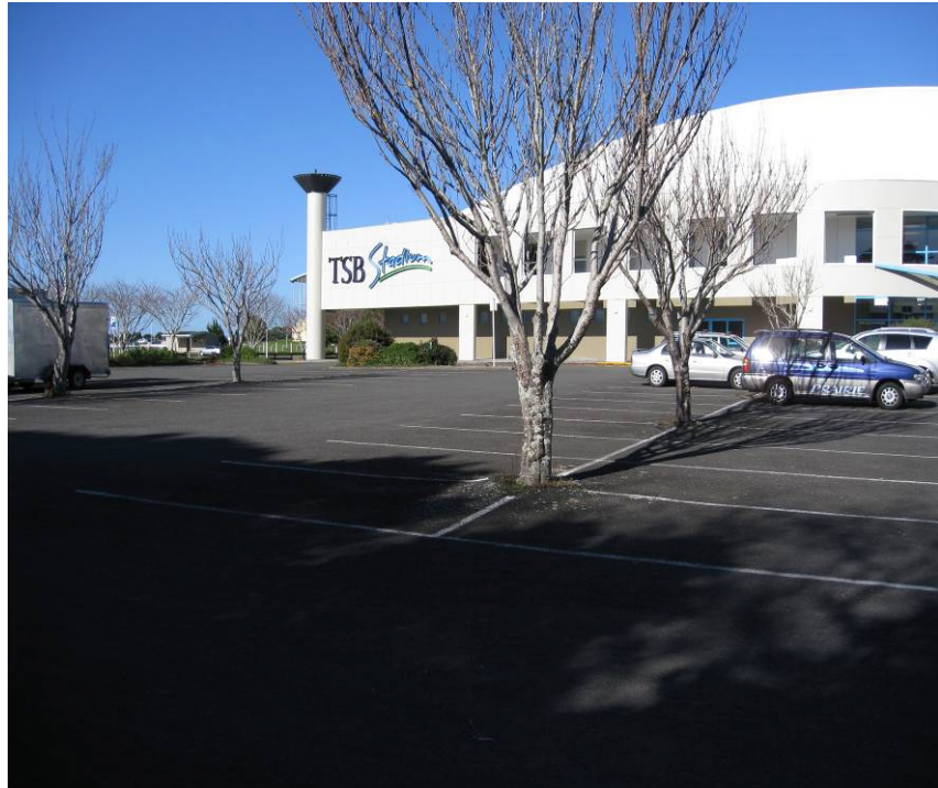
Photograph 2: TSB Stadium and Car Park
